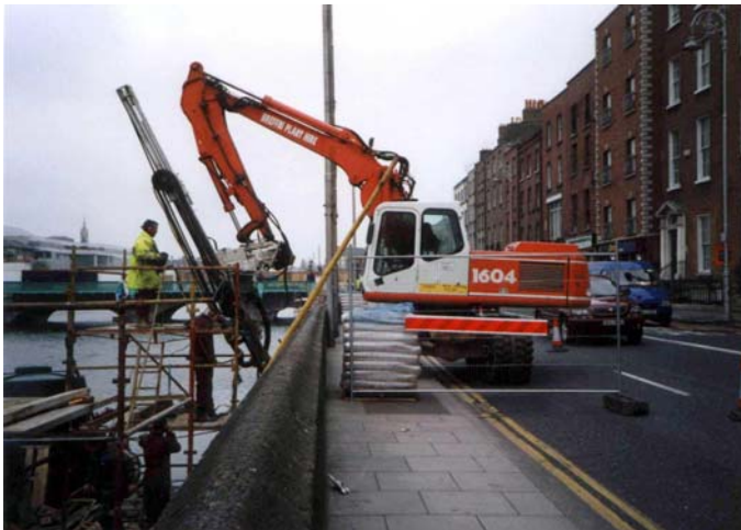
“Ischebeck” – Anchor drilling
